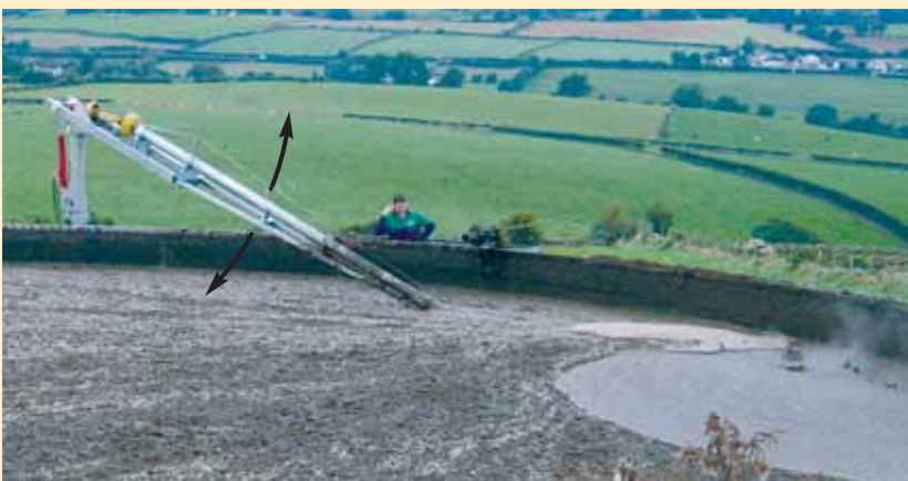
Complete homogenisation in a slurry tank with 44 m of diameter.
